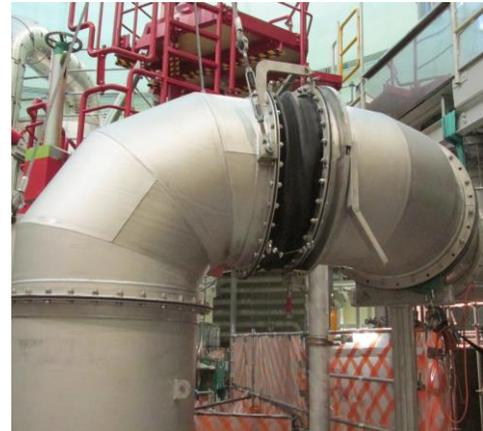
*Quick Disconnect Ductwork Connection*
