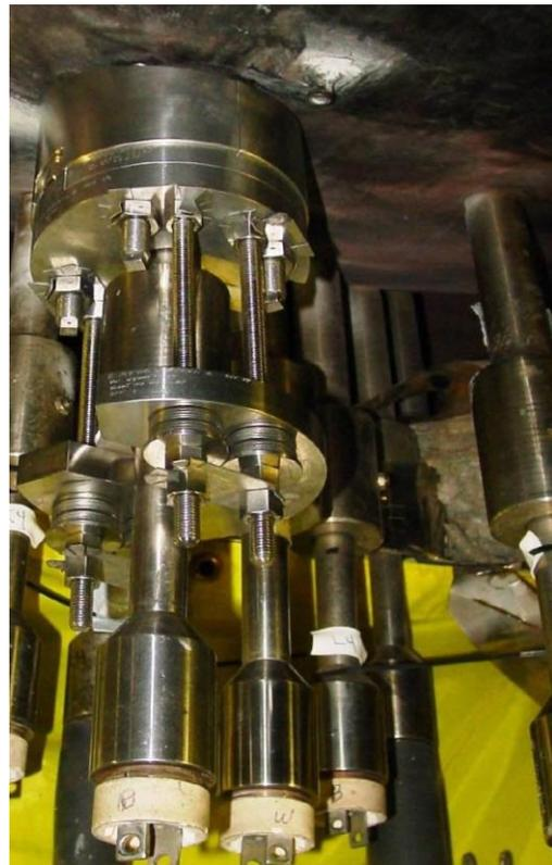
*MNSA Installed on Pressurizer Heater Sleeve*
