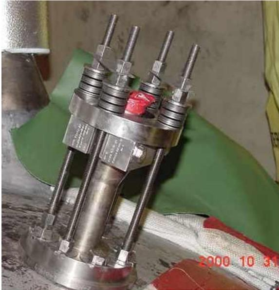
*MNSA Installed on RCS Piping Instrument Nozzle*
