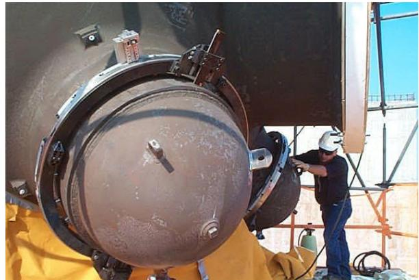
Outer diameter mounted pipe lathe shown installed on a replacement steam generator for severance cutting of the hydrostatic test cover
