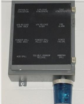
The Chemical Area Hazard Warning System (aka Blue Light System) is a rotating blue light beacon with an illuminating message panel.
